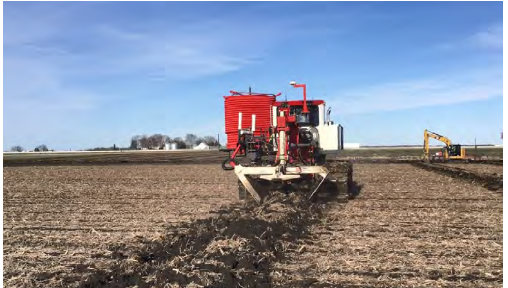
Figure 1. Tile Installation
