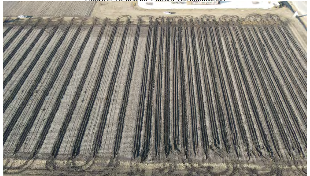
Figure 2. 15' and 30' Pattern Tile Installation
