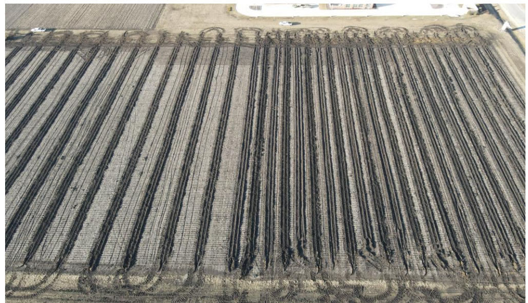
Figure 2. 15' and 30' Pattern Tile Installation
