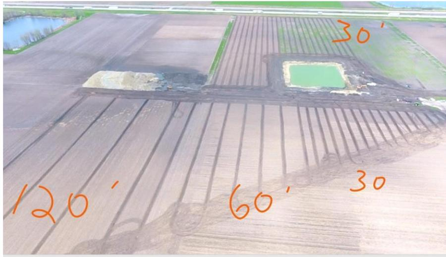
Water mains were installed around the farm reservoir to then collect and direct water from our new tile system into a station designed to “lift” water from the drainage system and deposits water to fill the reservoir.
